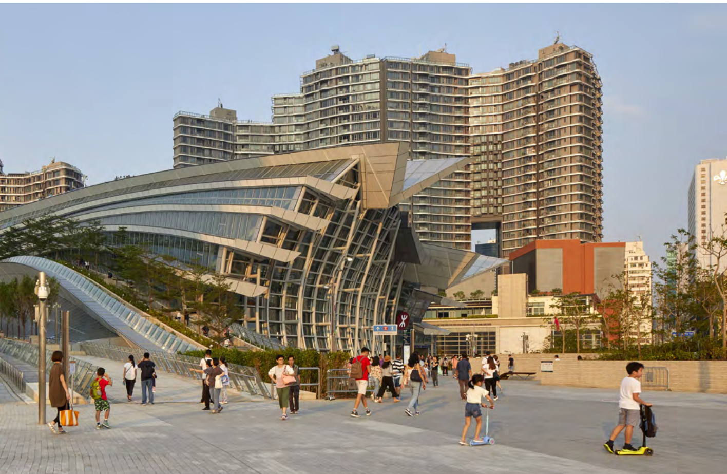
Hong Kong West Kowloon Station (Photo by Edmund Sumner)
